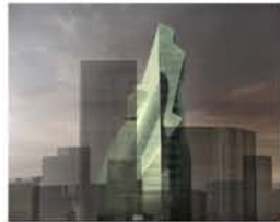
232. Tower Milan, Italy 2007-
