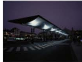
84. Bus Terminal Tours, France 1990–1992
