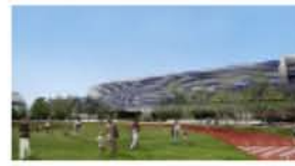
164. Barcelona Stadium Barcelona, Spain 2001*
