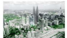
215. DNP Tower Kuala Lumpur, Malaysia 2005-
