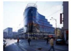
120. Andel Building Prague, Czech Republic 1995–2001
