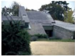
1. Delbigot Residence Villeneuve sur Lot, France 1970–1973
